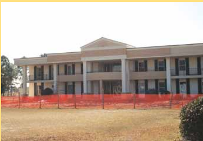
Ashby/Jones Halls renovation
